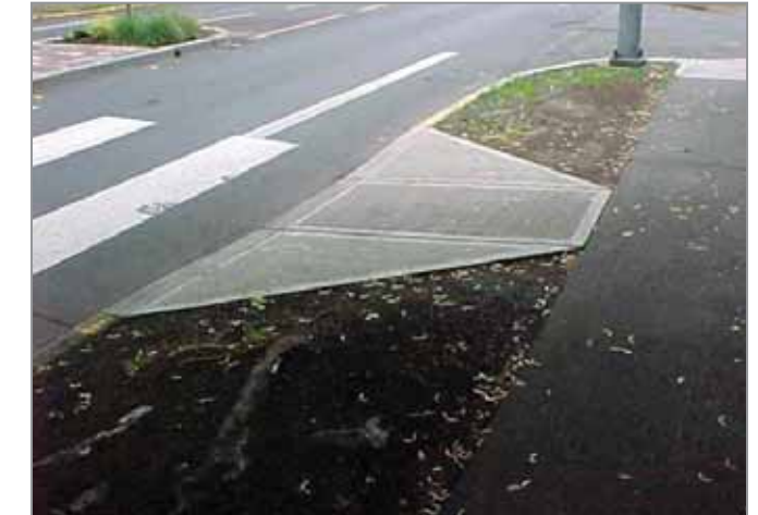
Ramps shall not exceed a 1:12 slope.
