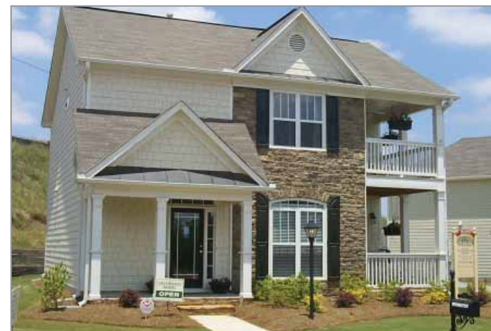
✗ Building wall materials may be combined on each facade only horizontally, with the heavier material below the lighter material
