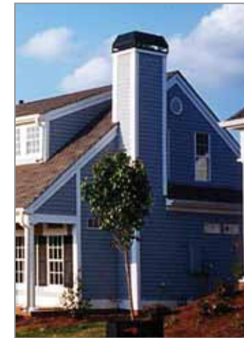
✗ Chimneys shall not be faced with siding.
