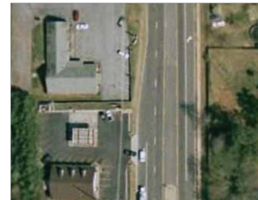
BUILDING + PARKING + STREET
