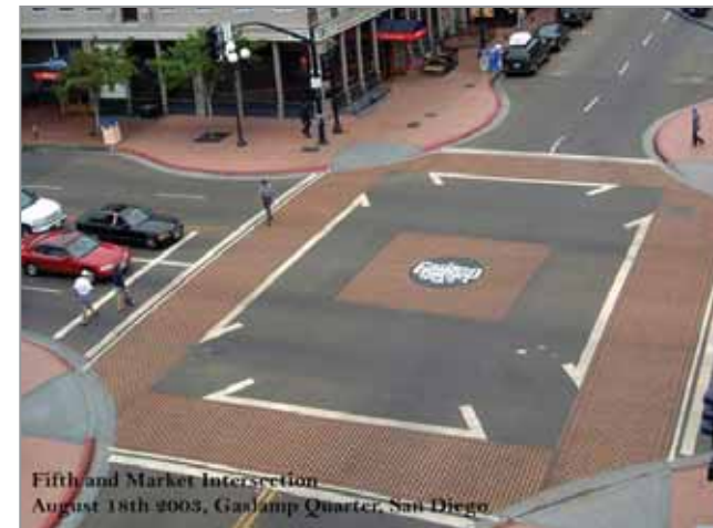
Inlaid colored asphalt crosswalk on Primary Streets
