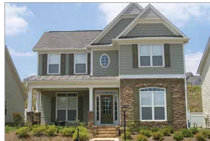
✓ Building wall materials may be combined on each facade only horizontally, with the heavier material below the lighter material
