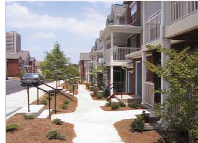
✗ There is no ramp from walkway to residence entrance
